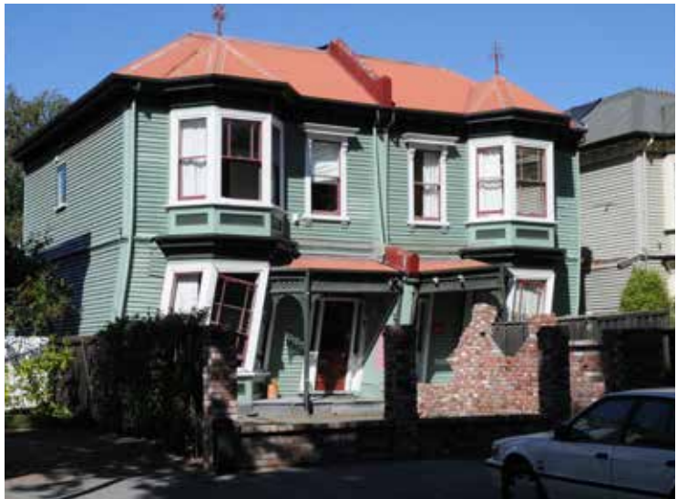
This turn-of-the-century wooden residence sustained major damage when it moved off its foundation during an earthquake.
