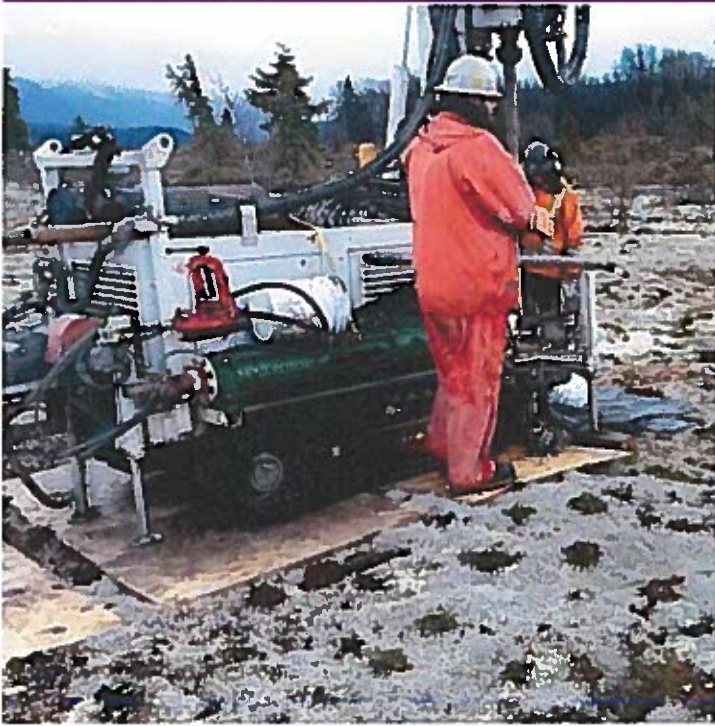
Small tracked drill rig mobilized on plywood.
